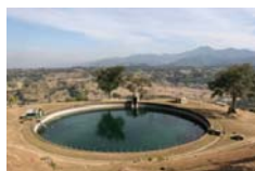
500 kW Pharping hydropower, 1911
