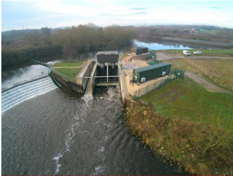
The 260kW Thrybergh project is one of two hydro projects to have been co-located with a 1.2MW/1.2MWh battery. Image: Barn Energy.
